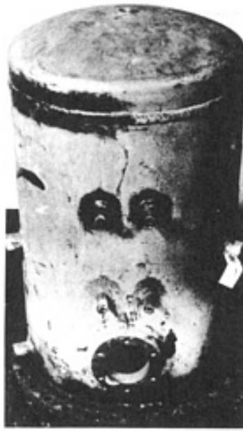
FIG. 9 AS-WELDED TYPE 430 STAINLESS STEEL SATURATOR TANK USED IN THE MANUFACTURE OF CARBONATED WATER THAT FAILED AFTER 2 MONTHS OF SERVICE. THE TANK WAS SHIELDED METAL ARC WELDED USING TYPE E308 FILLER METAL. SOURCE: REF 34
